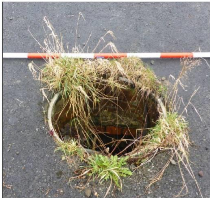
Plate 4.13: Man-hole with red-brick lining in former recreation area
