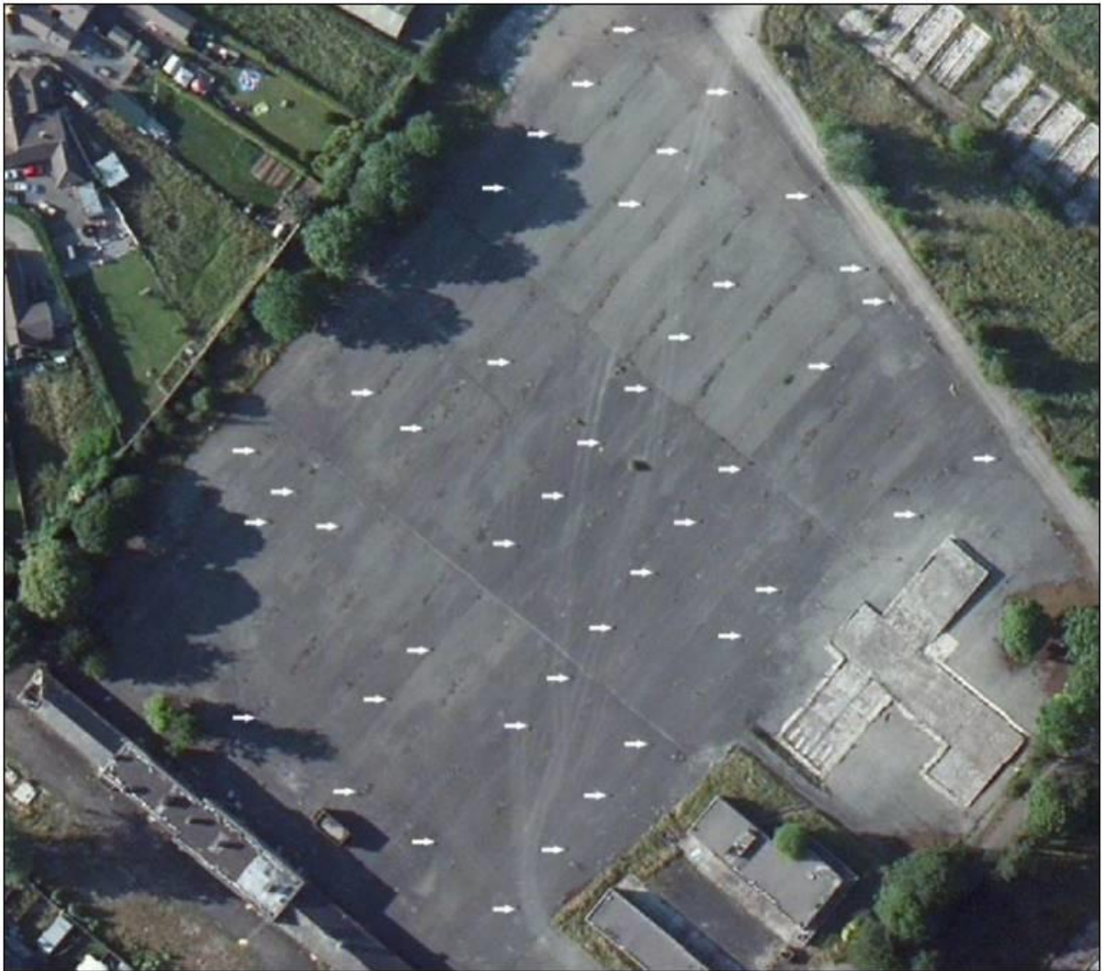
Fig. 4.15: Inspection / access manholes in former recreation area (those visible in aerial imagery are indicated by white arrows)
