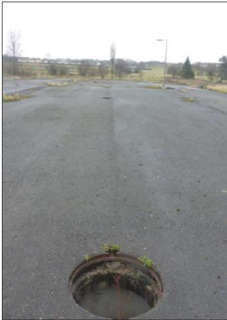
Plate 4.12: Line of man-holes in former recreation area, facing northeast
